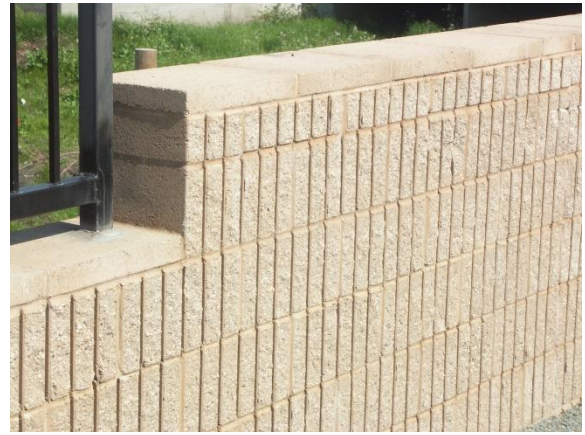
Photo 2: Close-up of Existing (Phase I) floodwall.
