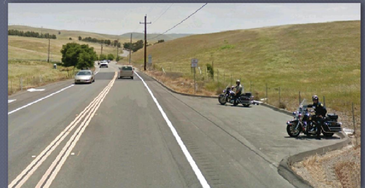
Safety/Enforcement Pull-Out Area
