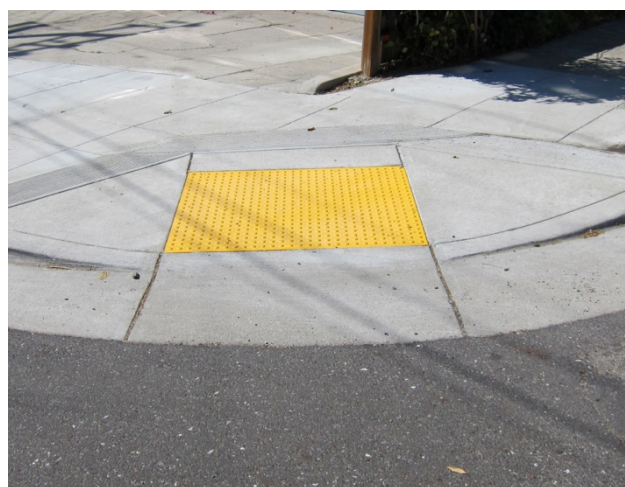
Figure 4-3: Curb ramp with detectable warning strip
